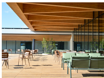
① CREVA VIEW TERRACE
