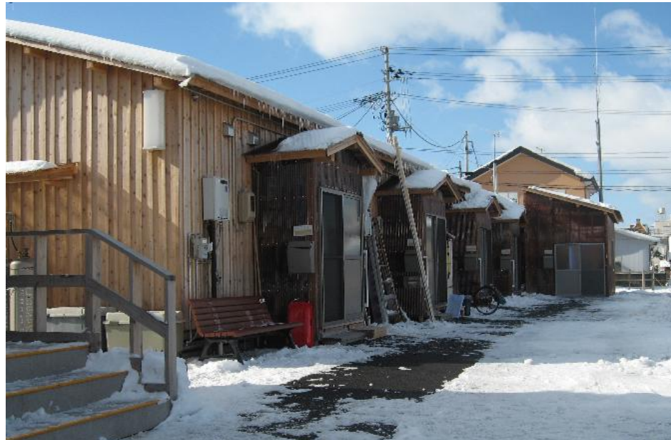
temporary housings in Aizu Wakamatsu City
